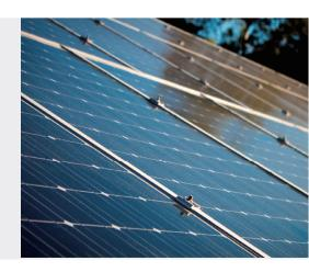
During operation of modules, there shall be no environmental factors to shade modules fully or partially. These environment factors including other modules, module mounting system, birds dwelling, dust, soil or plants. These will significantly reduce output power. LONGi suggests that the module surface should not be shadowed in any case.
